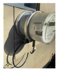
ConnectDER Solar Meter Socket Adapter All Versions of V5.2
