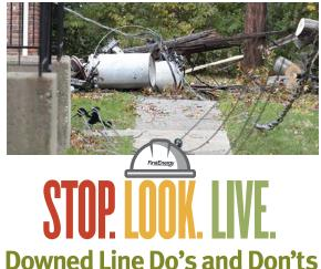
Severe weather and vehicle accidents can cause power lines to fall. Always assume downed lines are energized
