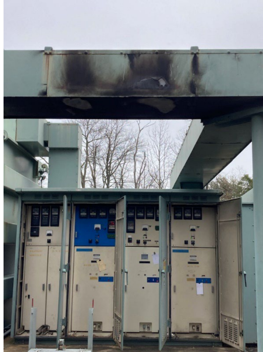
Figure 25: Monmouth Substation arcing event
