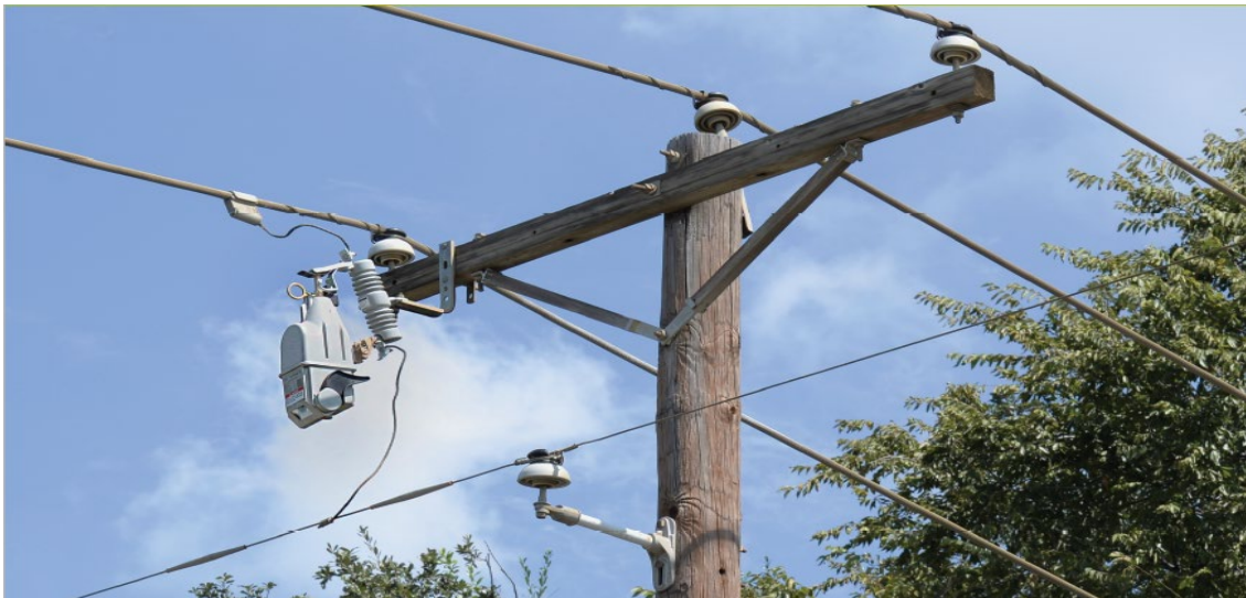
Figure 13: TripSaver II – Field Installed Device
