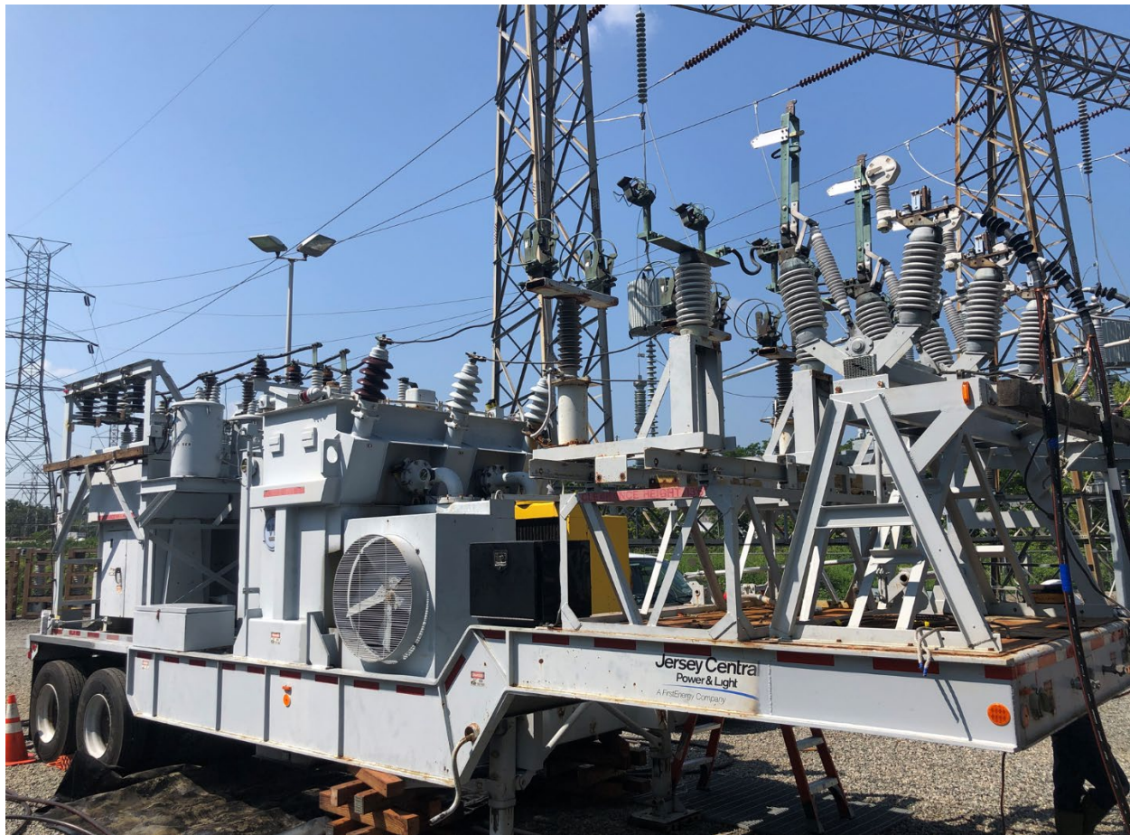
Figure 26: Recent Emergency Mobile Substation Installation
