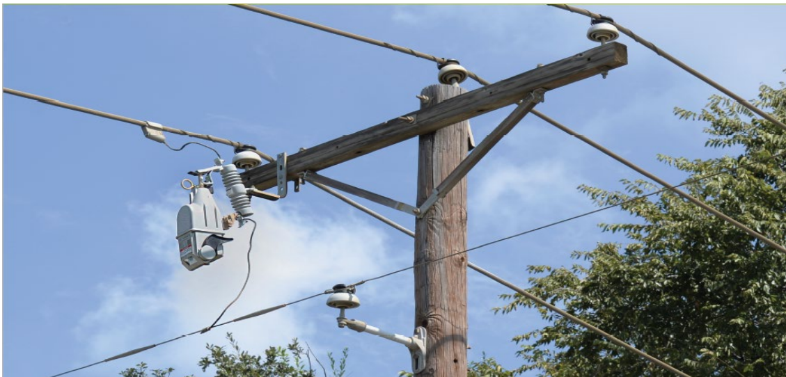
Figure 13: TripSaver II – Field Installed Device
