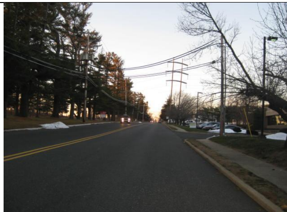
Northwesterly View along Green Grove Rd.
