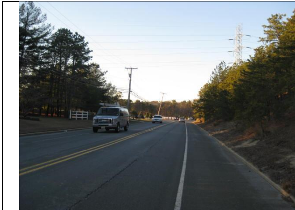
Northwesterly View along Herbertsville Rd.
