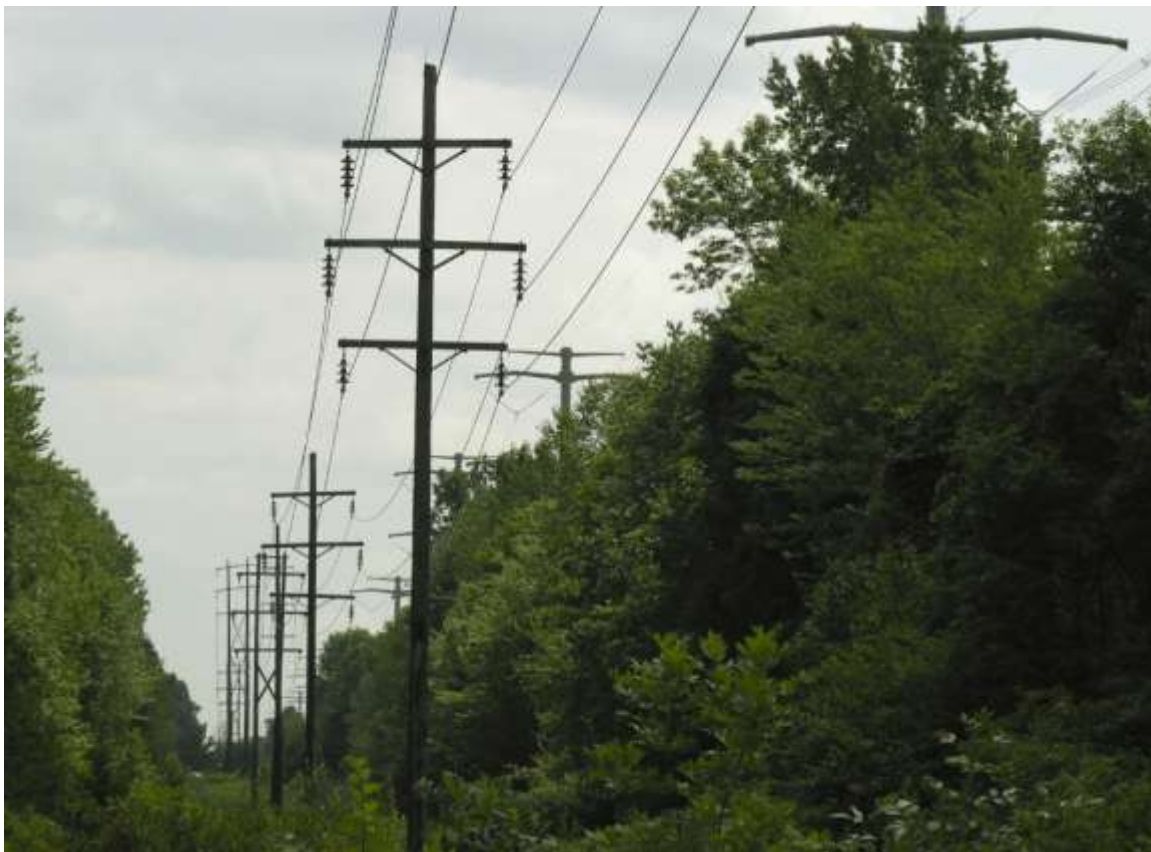
Figure 31 – Photograph looking south of electric and magnetic field measurement location along Miller Lane in Montville Township at approximately 2:20 PM on August 8, 2014 (corresponding to Table 10).
