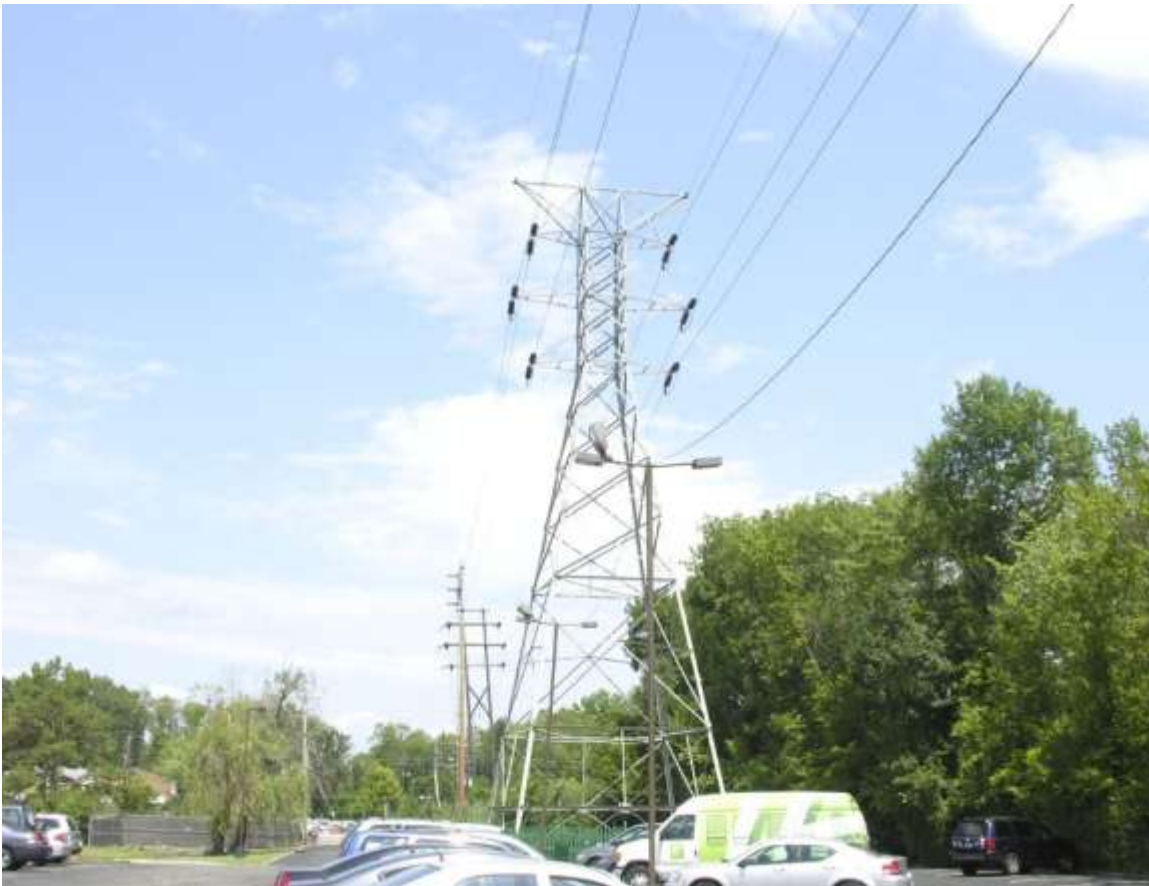
Figure 28 – Photograph looking north of electric and magnetic field measurement location along Route 46 in Parsippany-Troy Hills Township at approximately 1:15 PM on August 8, 2014 (corresponding to Table 7).
