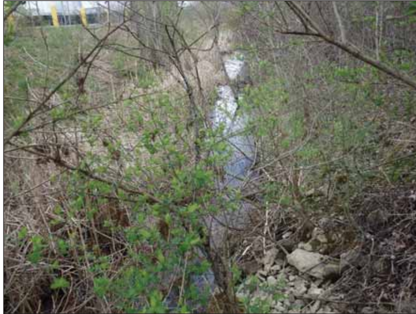
Photograph 9. View facing east facing downstream along Stream 0423-04
