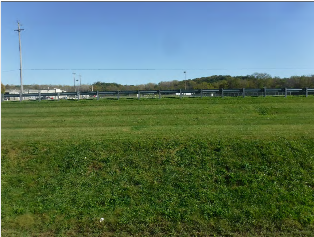
Photograph 4.4. Overview of Project Area at SL A129, facing east.
