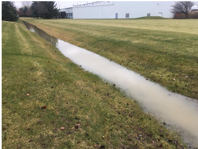
Photograph 4: Stormwater Drainage Feature south of State Route 795 facing east. (December 21, 2018)
