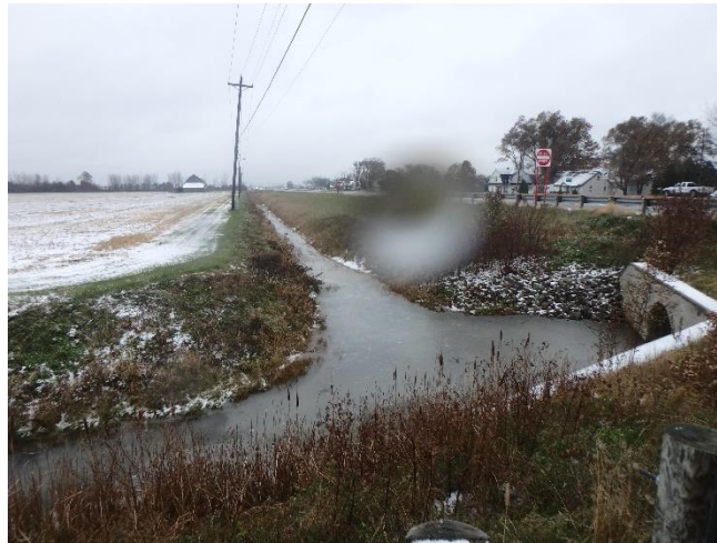
Photograph 2. Stormwater drainage feature along State Route 795 facing west. (November 15, 2018)
