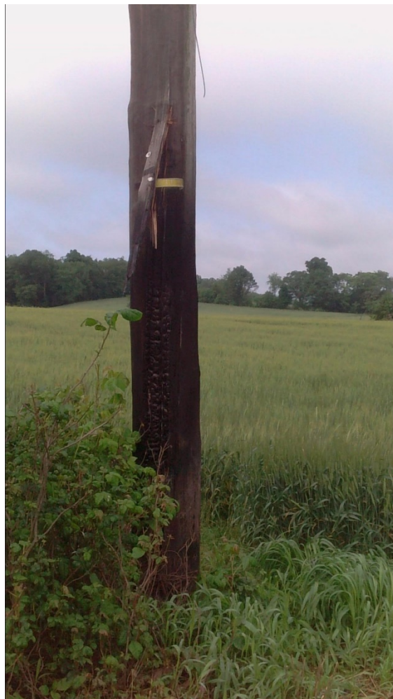
Photograph 5: Pole fire and broken-down ground
