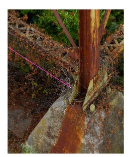
A 2024 iHawk Steelworks drone inspection was completed to confirm the severity of the deterioration on all three towers. Using the National Grid grading system, iHawk ranked all steel members on a scale from 1-6. See Table 1 for grading information. See Table 2 for the tower results. A majority of the members (58%) were graded as 4, confirming that most members are significantly corroded and/or pitted. Around 1% of members were
