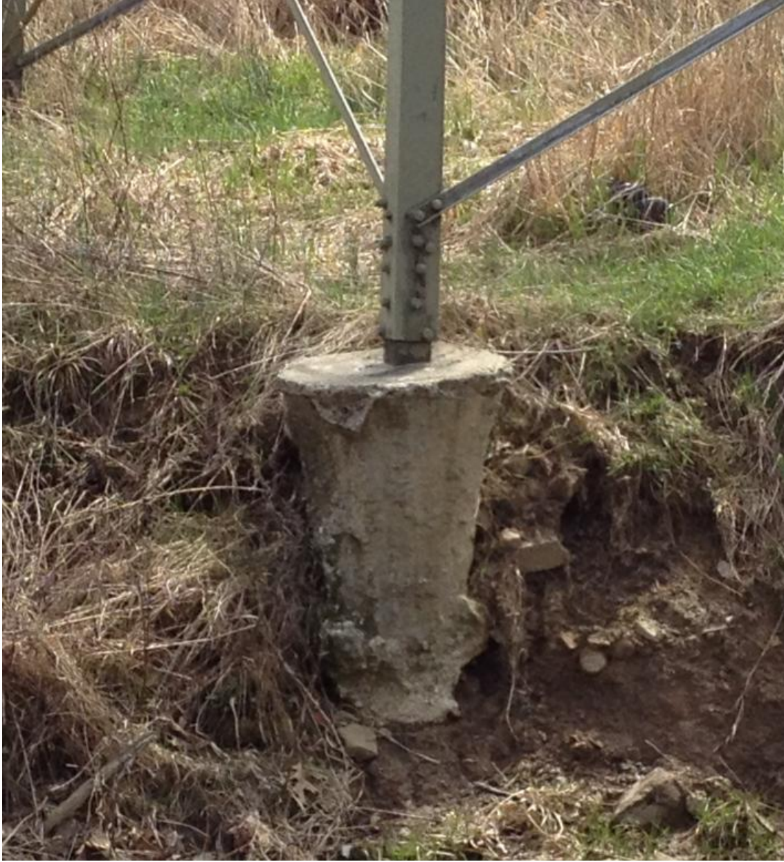
Photo 3. Exposed tower leg foundation.
