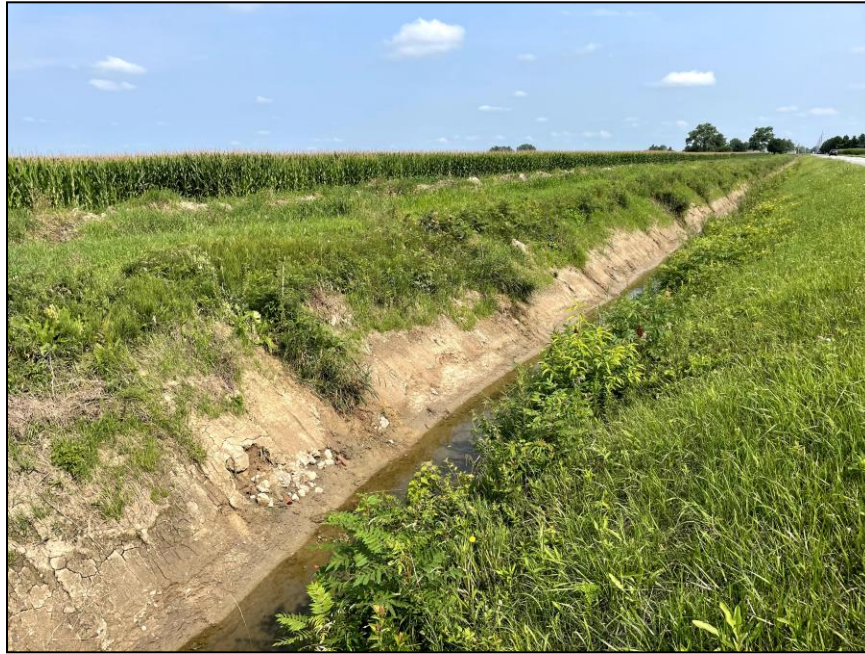
Photograph 3: Facing north looking downstream along Stream 3.
