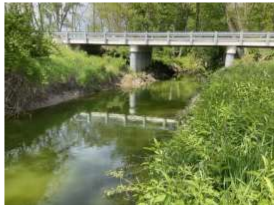
Photograph 4. SOH-KLV-001, Upstream Facing West (05/12/26)
