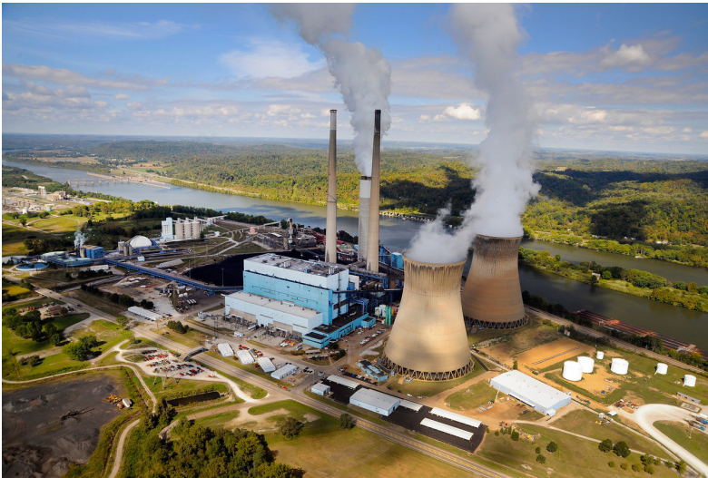
Pleasants Power Station is located in Willow Island, West Virginia, along the Ohio River.
